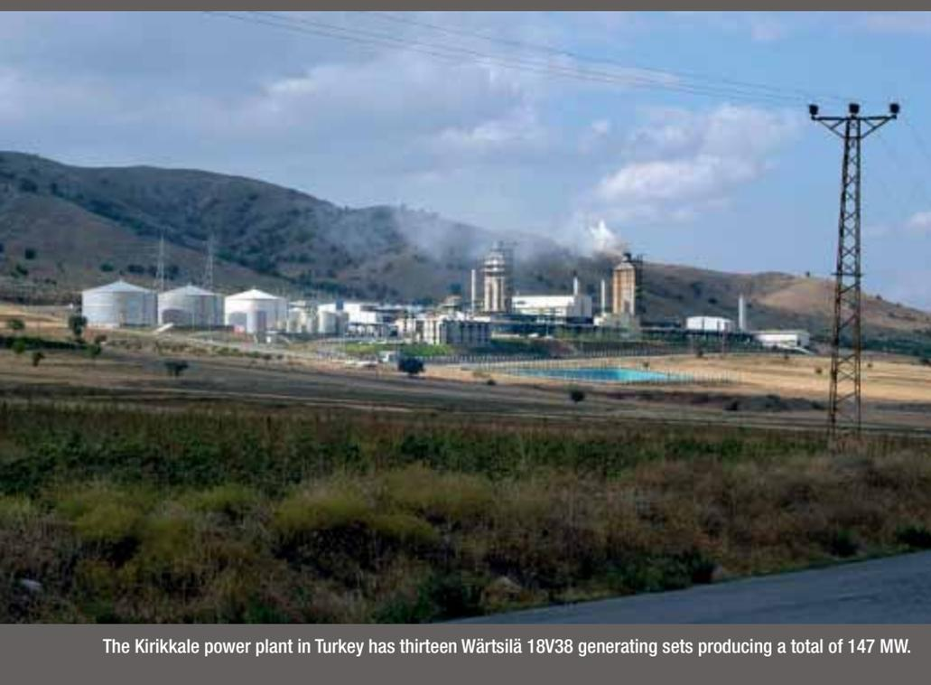
The Kirikkale power plant in Turkey has thirteen Wärtsilä 18V38 generating sets producing a total of 147 MW.
